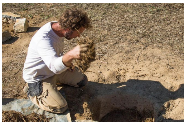
Figure 19. A mixture of straw and humid soil is placed above
