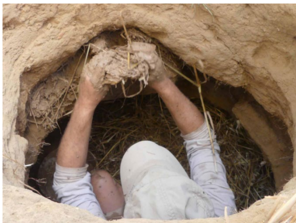
Figure 16. Straw is placed on the wall of the silo
